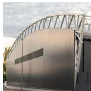
Sandwich Panel Rigid steel sides with a polyurethane or rock wool core for thermal and acoustic insulation.
